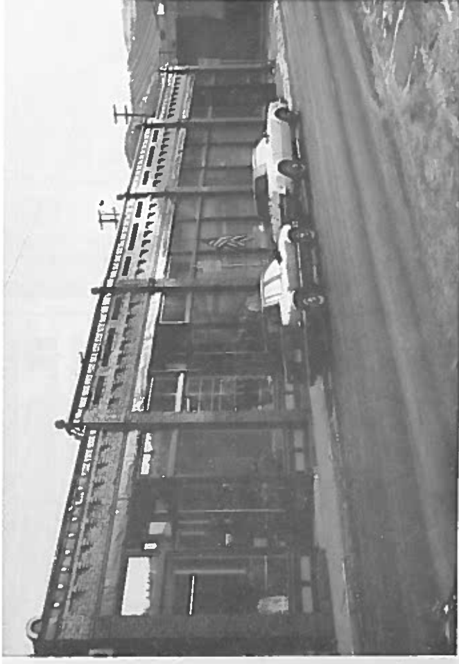
(Left Below) The C.W. Cannon Building after rehabilitation. Original sized windows are restored complete with transoms. The brick facade has been cleaned and painted. Decorative features of the building cornice have been emphasized by the creative use of color. Bright afternoon sunlight is controlled by mini-blinds. The storefront rhythm is restored without altering the interior use.
