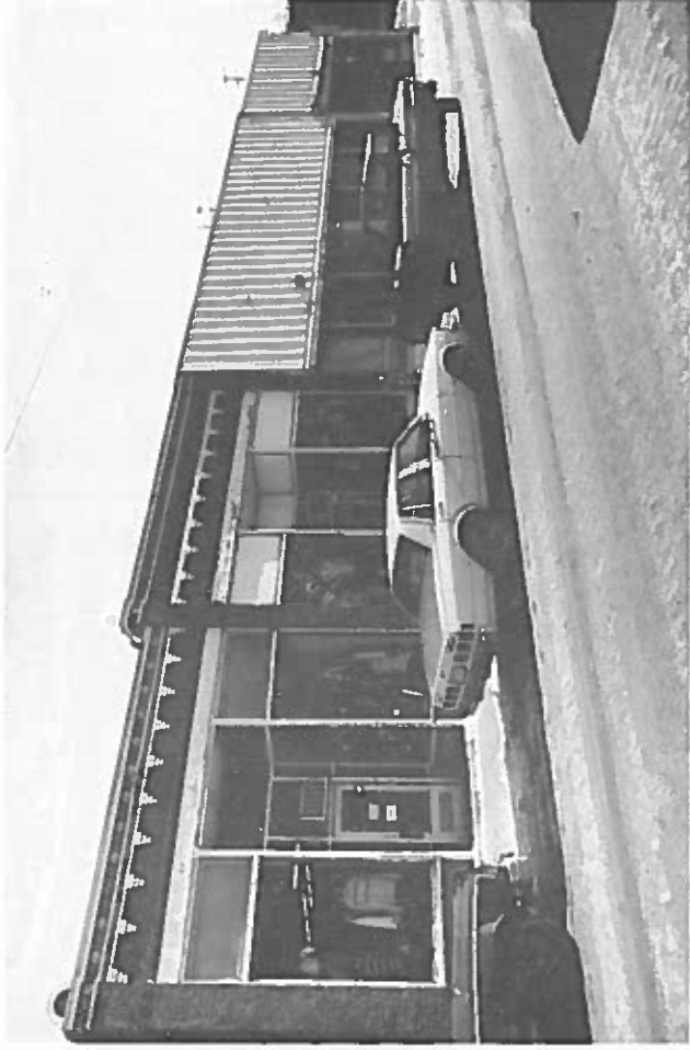
(Left Above) The C.W. Cannon Building before rehabilitation. The far right bay of the building had been "modernized" with a sheet metal false front. The rhythm of the building facade was disrupted and many historical details lost. Transoms were covered, permanently restricting the natural light.
